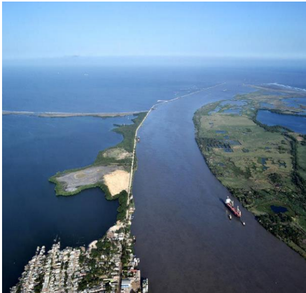
Figure 11 - Location of protective structures at the beginning of the access channel to the Barranquilla port in Colombia
