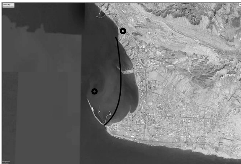
Figure 9- Coastline changes because of primitive construction breakwater
