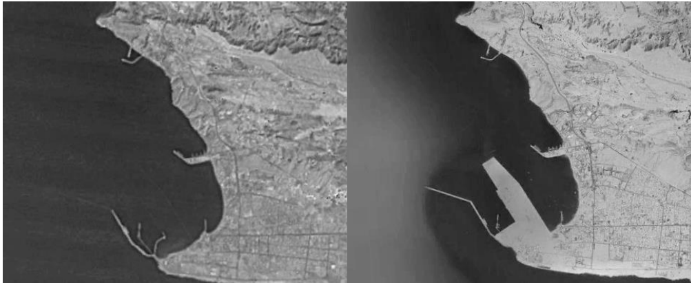
Figure 7- Construction of breakwater at eastern part of Chabahar bay. (Left): first construction, (Right): harbor extension.
