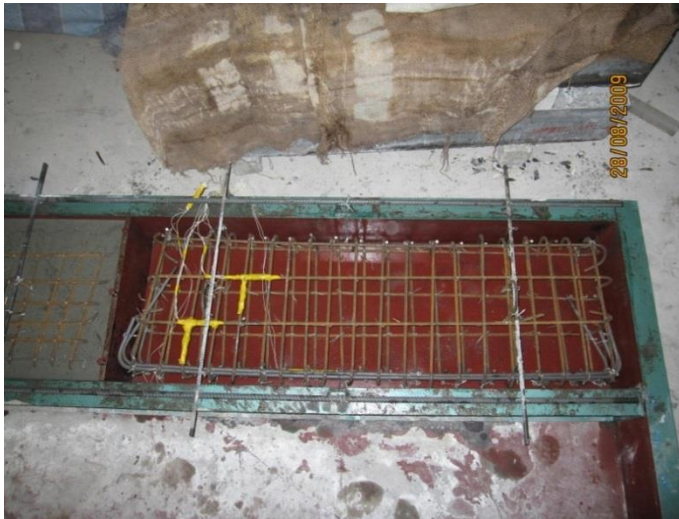
Figure 2: The casting arrangement and deep beam fabrication
