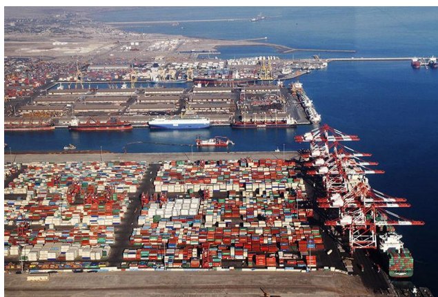
Figure 2. Aerial view of Shahid Rajaei Port
