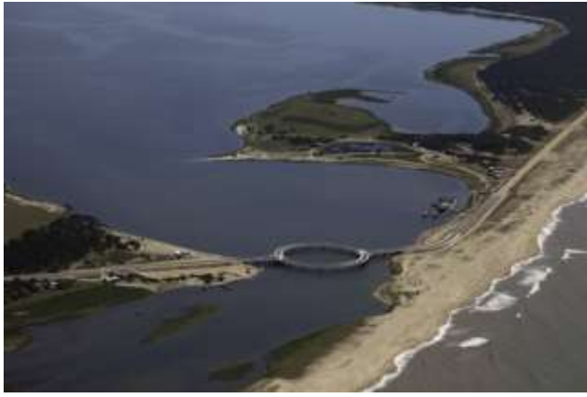
Figure 1: A coastal curved bridge (Laguna Garzon bridge in Uruguay).
