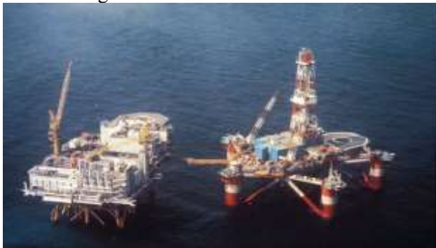
Figure 1: oil platform in the North Sea called Alexander The sedco135 semi-submersible drilling rig, which started its activity in the Gulf of Mexico in 1965, suffered failure due to fatigue in one of its braces after two years in 1967.
