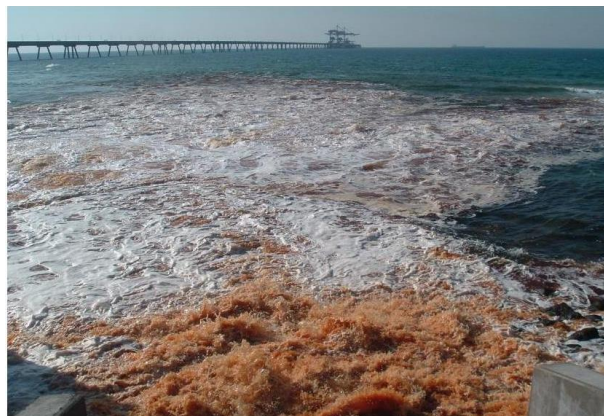
Figure 13- Effluent from the discharge of effluents from the surface desalination system in Ashkelon (Jirka, 2003 and 2004).
