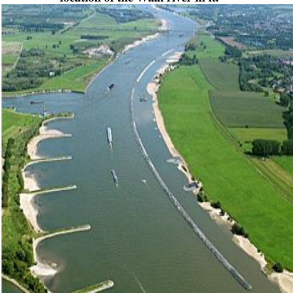
Figure 2- The picture of the Waal river and the vertical breakwater structures in the outer arch and the middle wall in its inner arch
