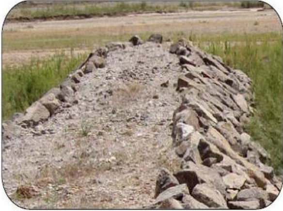
Figure 9- View of a constructed spillway in the Qezel Ozen-Qowijan River
