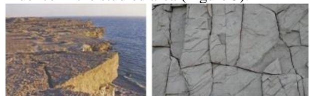
Figure 5. Faulted and jointed cliff coasts, Tis and Lipar coastal areas
